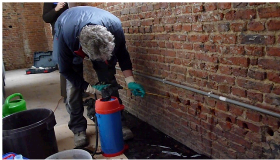
Figure 4. Impregnation without pressure
