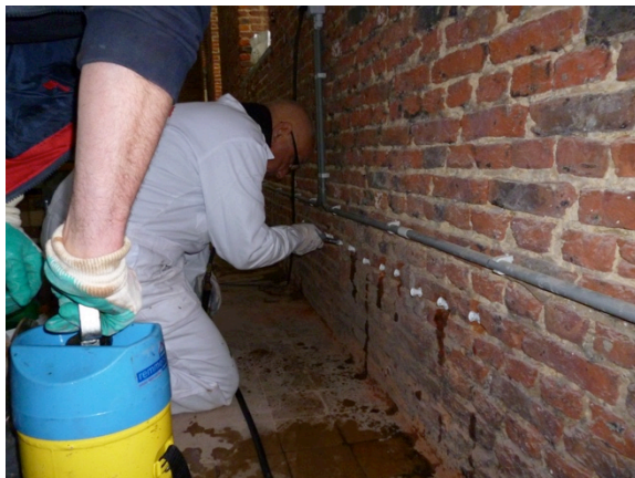
Figure 5. Injection with pressure
