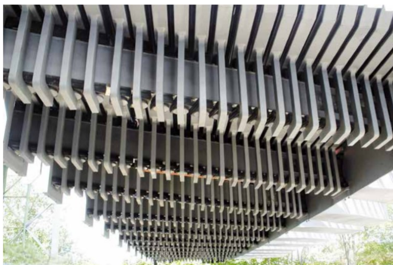
Figure 73 - Seismic lamella joint [38]
