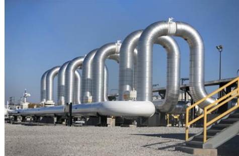
Figure 18 - U shaped pipe connection 5
