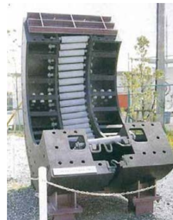
Figure 19 - Seismic joint of a circular tunnel 7
