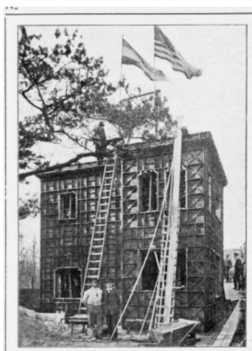
Figure 9 & 10 Cast concrete house in Santpoort, Architectura , 1911.
