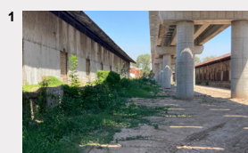
1 MR.01.BB.001 BOCA BARRACAS Components storage
