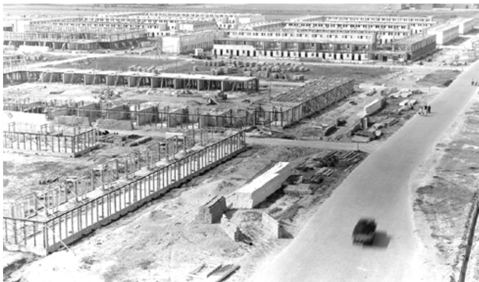
Figure 4. Nemavo-Airey system. Construction of the residential neighbourhood of Jeruzalem in Amsterdam (1950). Source: Stadsarchief Amsterdam.
