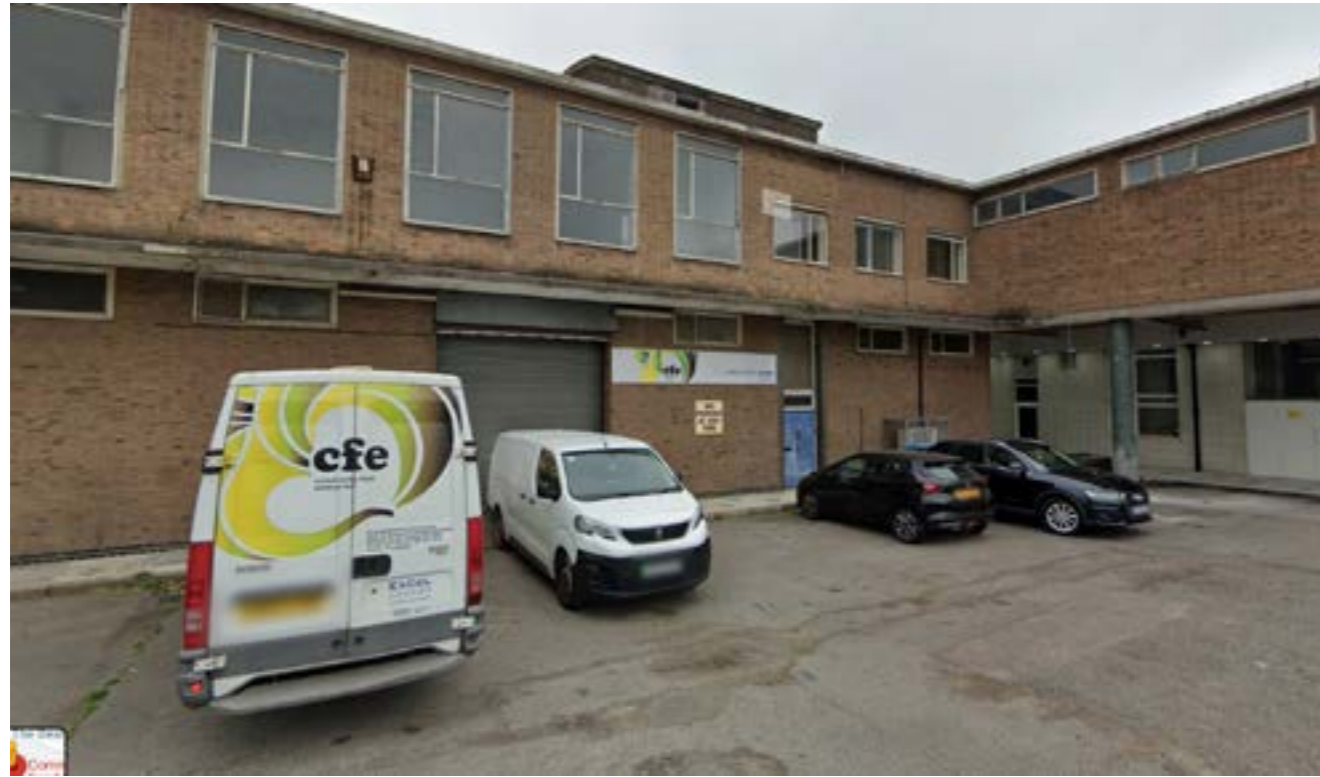
Figure 28: Dilapidated building that looks abandoned, accessed 05 May 2023, <Google maps>
