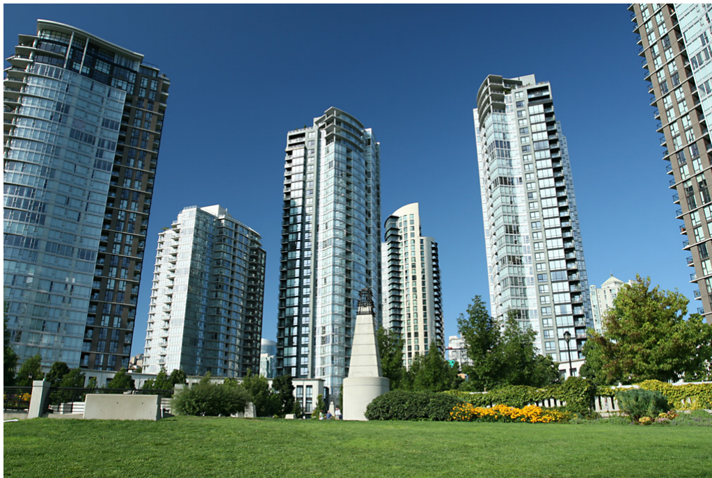
Figure V – High rise buildings, influences of project development in booming times
