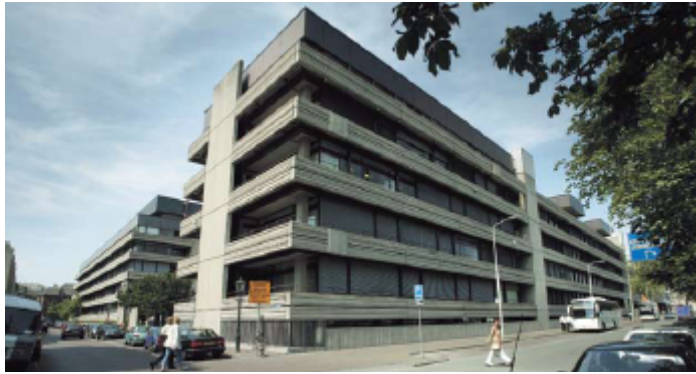
Figure 48- The finance building 1975
