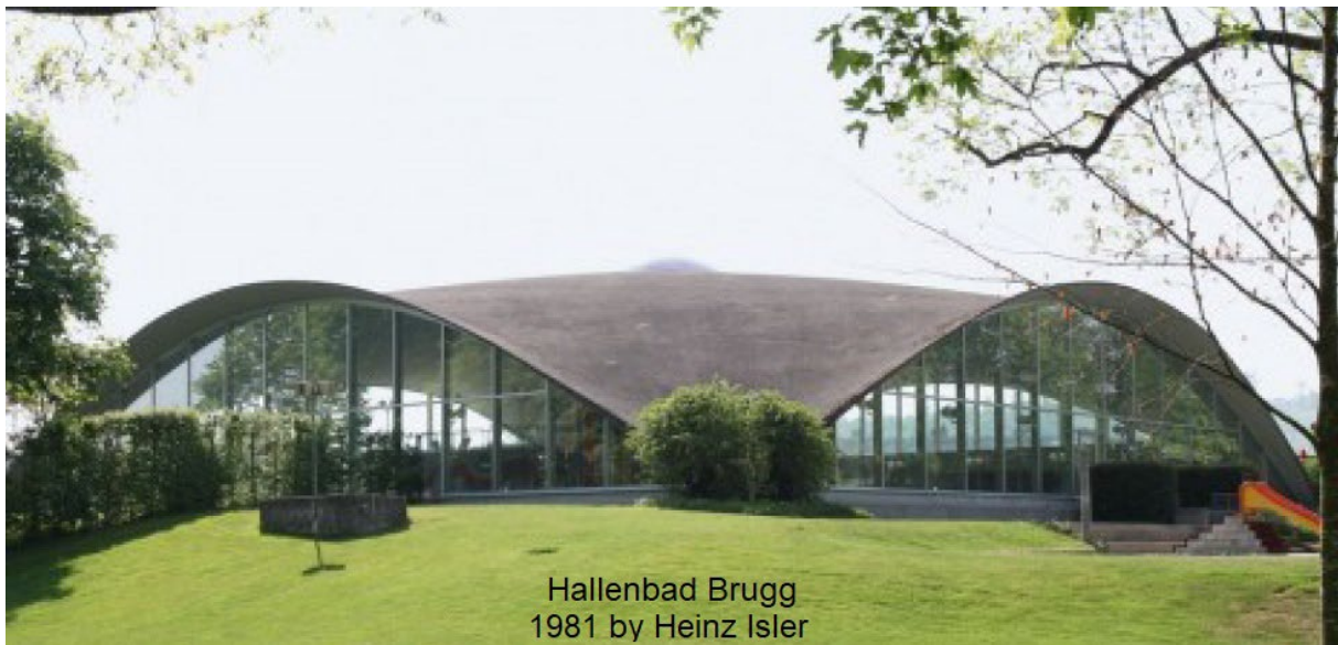
Figure 64 Hallenbad by Heinz Isler [image Peter Eigenraam]
