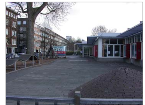
Fig. 46 | Primary school at Noorderhavekade
