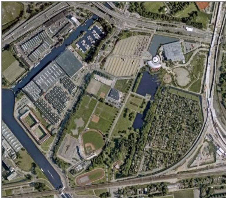
Fig. 151 | Situation in quadrant C (2009, Google Earth)
