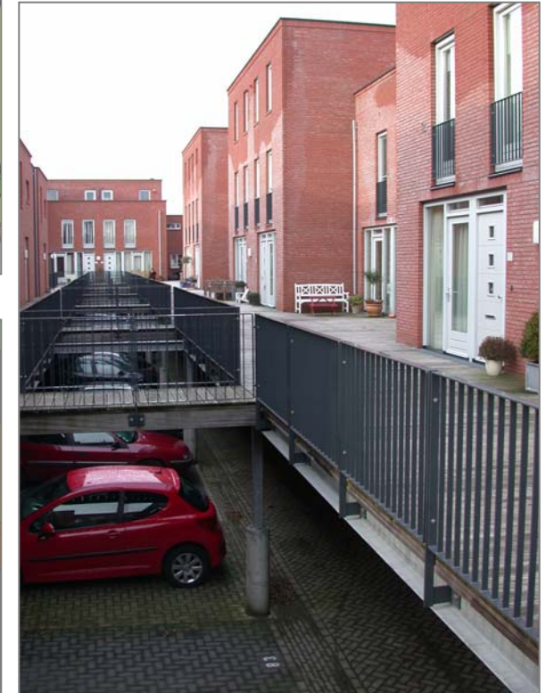
Fig. 119 | Parking and plank bridges in Den Bosch
