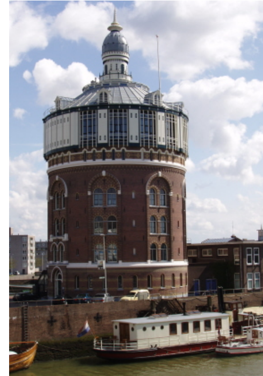
fig. 3 Water tower www.010.nl
