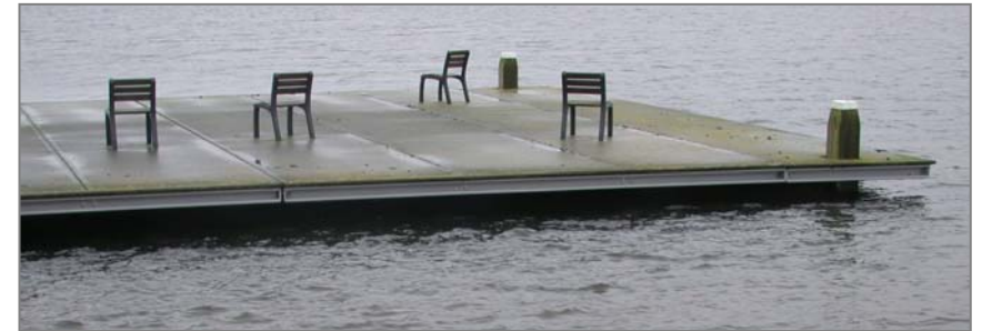
Fig. 175 | An example of a platform in the water (Zevenhuizenplas)
