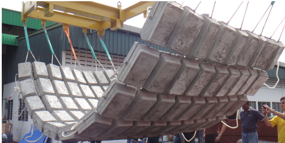
Figure 2.7: Articulated concrete block mattress (Siam Gabions, 2011)
