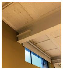
Figure 29: Steel I-beams are attached to brick columns.
