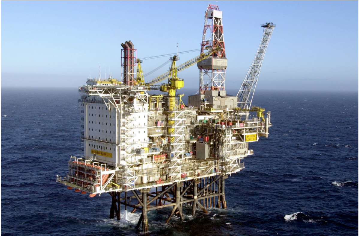
Figure 3.1: The Gyda topsides [retrieved from http://www.align.no/successful-gyda-project/ ]
