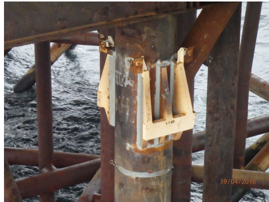
(b) An on-leg lift point
