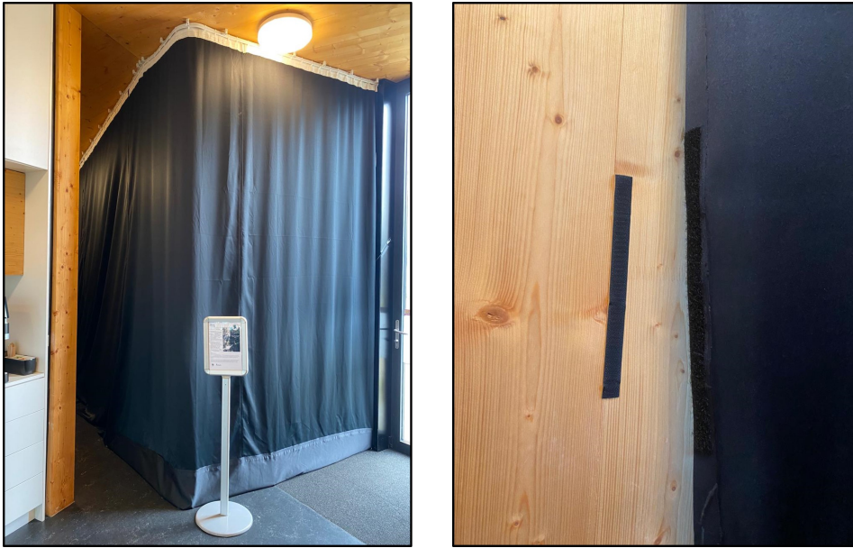
Figure 5.3: Curtain design (left) and velcro tape strategically placed to ensure complete enclosure of the lab space (right).
