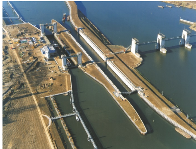
Figure A-2: Navigation lock in Lith, The Netherlands [24]
