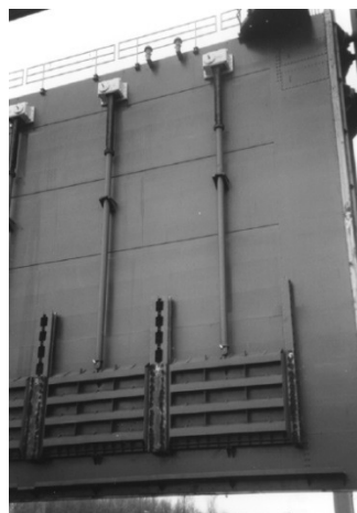
Figure A-9: One-sided retaining valve in a gate [24]
