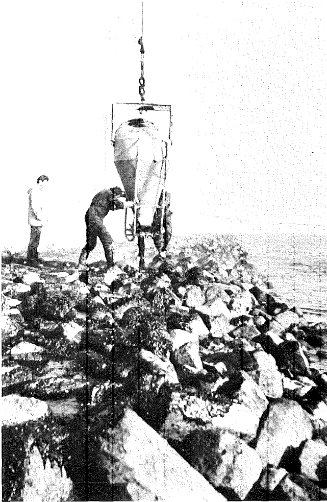
Photo 18 Grouting a crushed stone layer using a bucket
