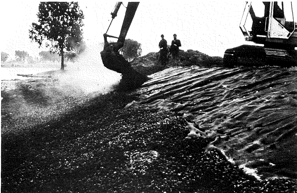
Photo 21 Placing an open stone asphalt layer on a filter cloth using a backhoe
