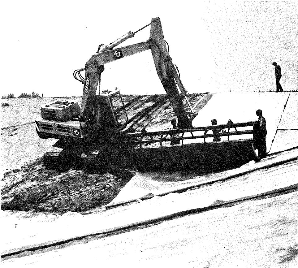
Photo 28 Placing a prefabricated membrane (Hypofors)
