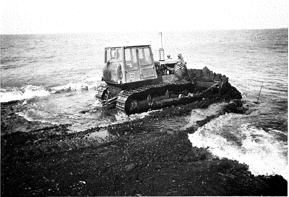
Photos 25, 26 Construction of a lean sand asphalt reclamation bund
