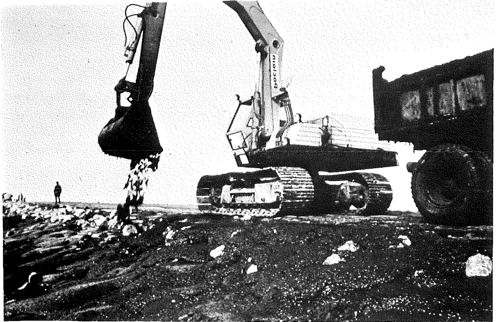
Photo 17 Grouting a crushed stone layer with the use of a crane
