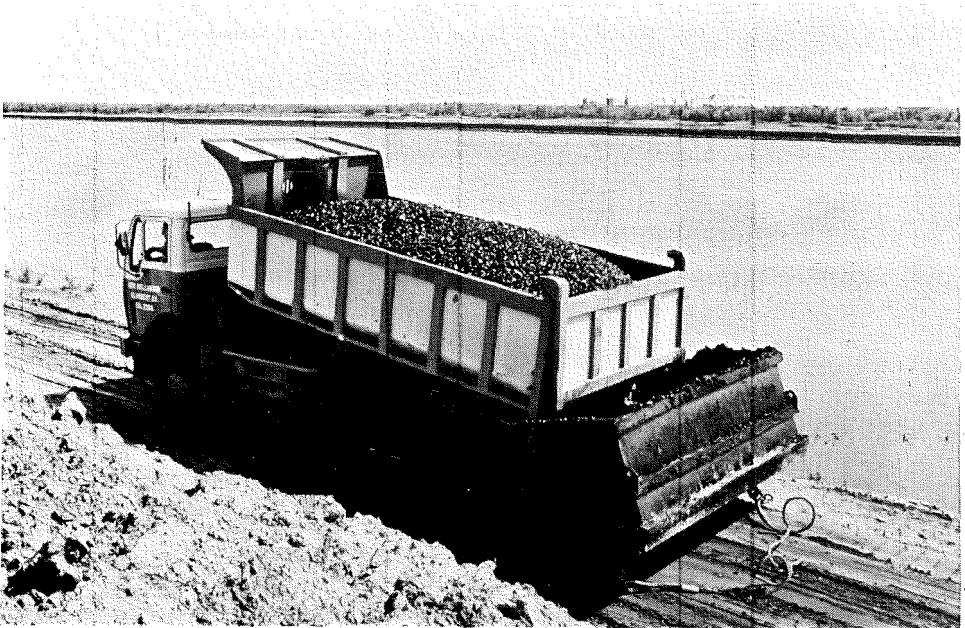
Photo 20 On site storage of open stone asphalt in a transport container
