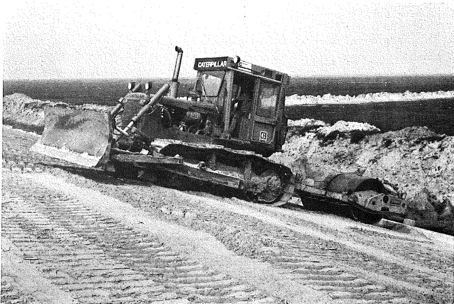
Photo 4 Compacting the sandbed using a vibratory roller
