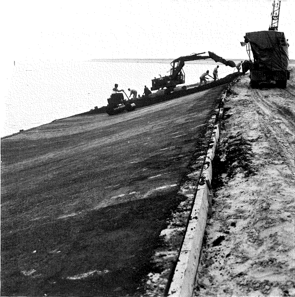
Photo 10 Construction of an asphaltic concrete revetment: The crane dumps the asphalt on the slope; the backhoe spreads the asphalt
