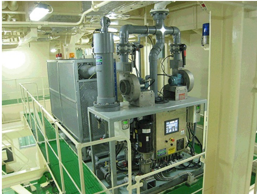
Figure 4.5: Balpure ballast water treatment system from De Nora [? ]
