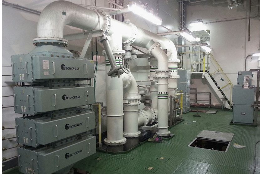
Figure 4.10: Electro-Cleen ballast water treatment system from Techcross [? ]
