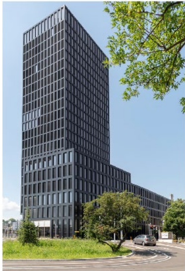
Building Integrated PhotoVoltaics (BIPV)
