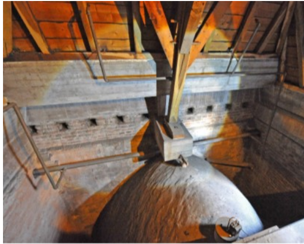
Figure B.9: Walls with concrete ring beam in the roof space of the stone vaults (from Nusselder and Zandijk, 2015)
