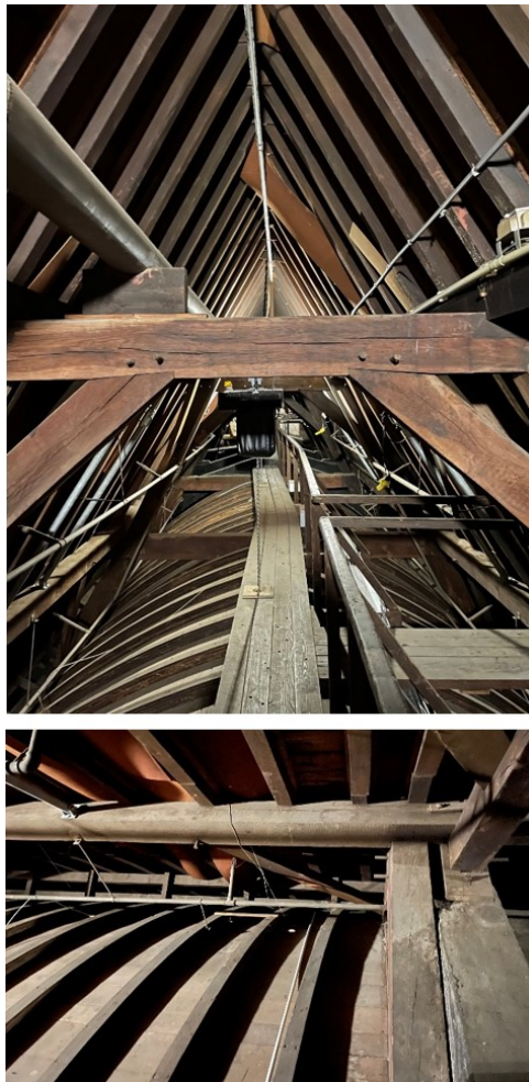
Figure B.10: Roof space wooden vault with walkway - limited space and roof structure with protective blankets against the entry of rain and snow
