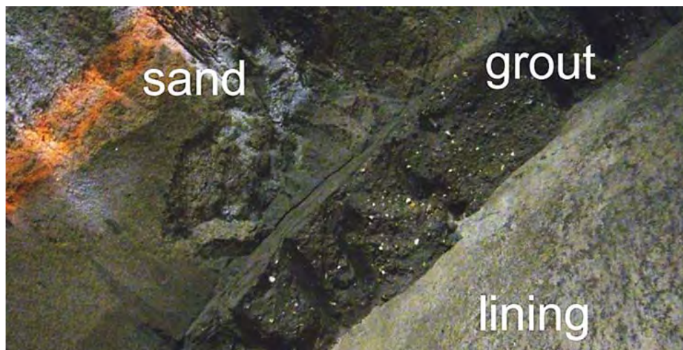
FIGURE 69: LAYER OF TAILVOID MORTAR (GROUT) [3]
