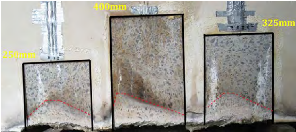
FIGURE 44: FLAME INTRUSION PATHS IN THE GAPS OF SAMPLE 2
