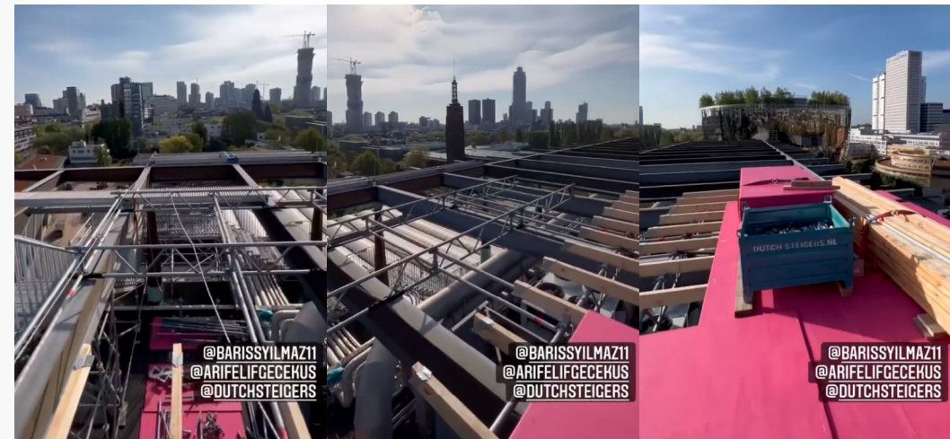
Lightweight timber frame with plywood covering fixed onto a low height steel truss sub-frame
