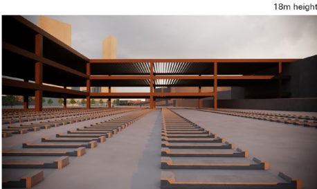
20m Grid: 20m span, 1200mm deep
