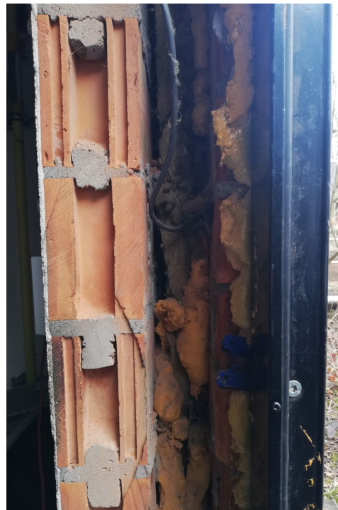
details of wall composition
