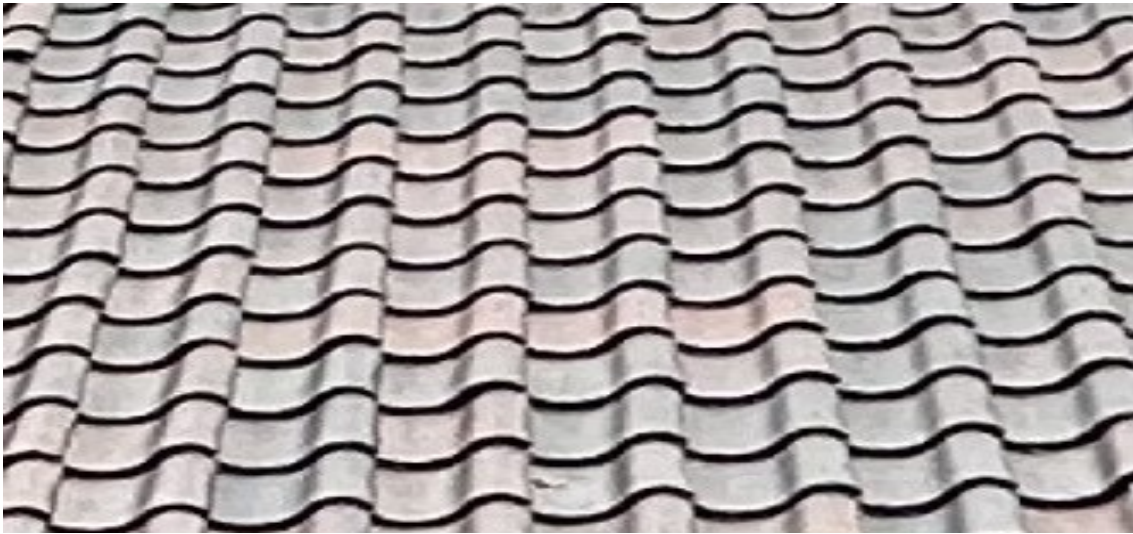
Figure 4.6: Reused roof tiles
