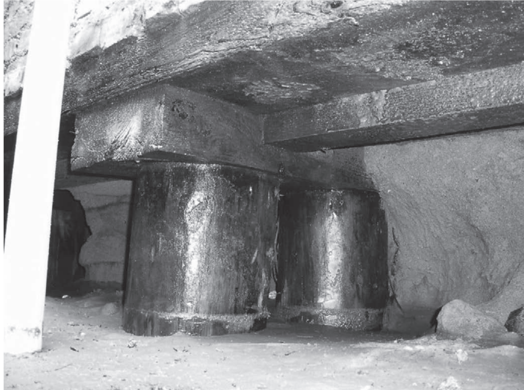
A commonly used foundation construction in the Netherlands of pile pairs, the so-called Amsterdam foundation type. Photo: Wooden foundation piles and its underestimated relevance for cultural heritage René K.W.M. Klaassen, Jos G.M. Creemers
