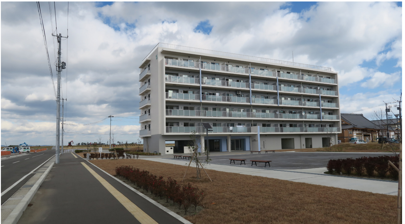
figure 80. Tsunami resilient apartments keep the ground floor free of housing units. Author
