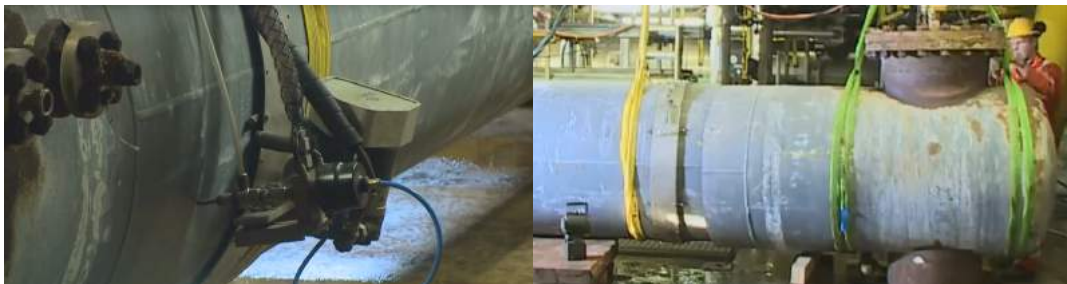
Figure 3.4: Piecemeal dismantling, state-of-the-art water jet cutting by the company Curved Cuts B.V.
