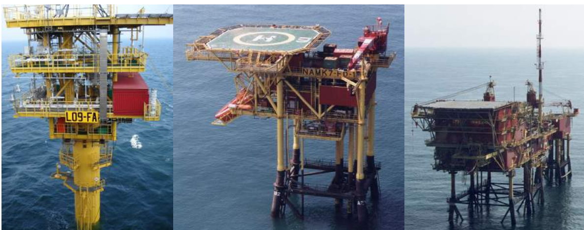
Figure 2.1: Typical ONEgas Assets; Monotower, Normally Unmanned Installation and Manned Installation
