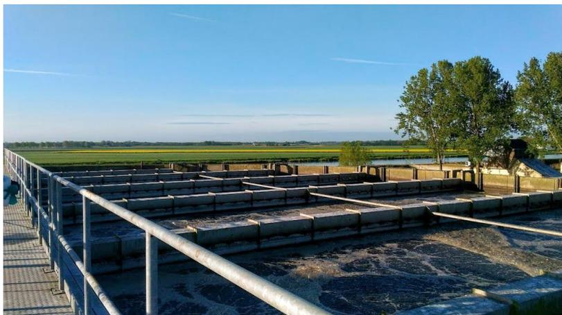
Figure 8: Nereda reactor in Garmerwolde during the aerobic reaction phase when sampling occurred.
