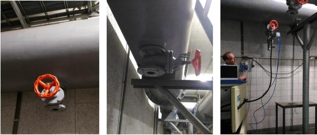
Figure 6: Sampling valve underneath the pressure main at the wastewater treatment plant. The installed on-line sampler (right) could not operate due to the elevated settling of suspended solids and the impossibility of installing a flushing mechanism due to the safety regulations for the basement of the WWTP.
