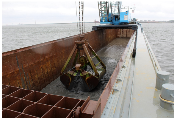
(a) Crane loading the mud into the hopper.
