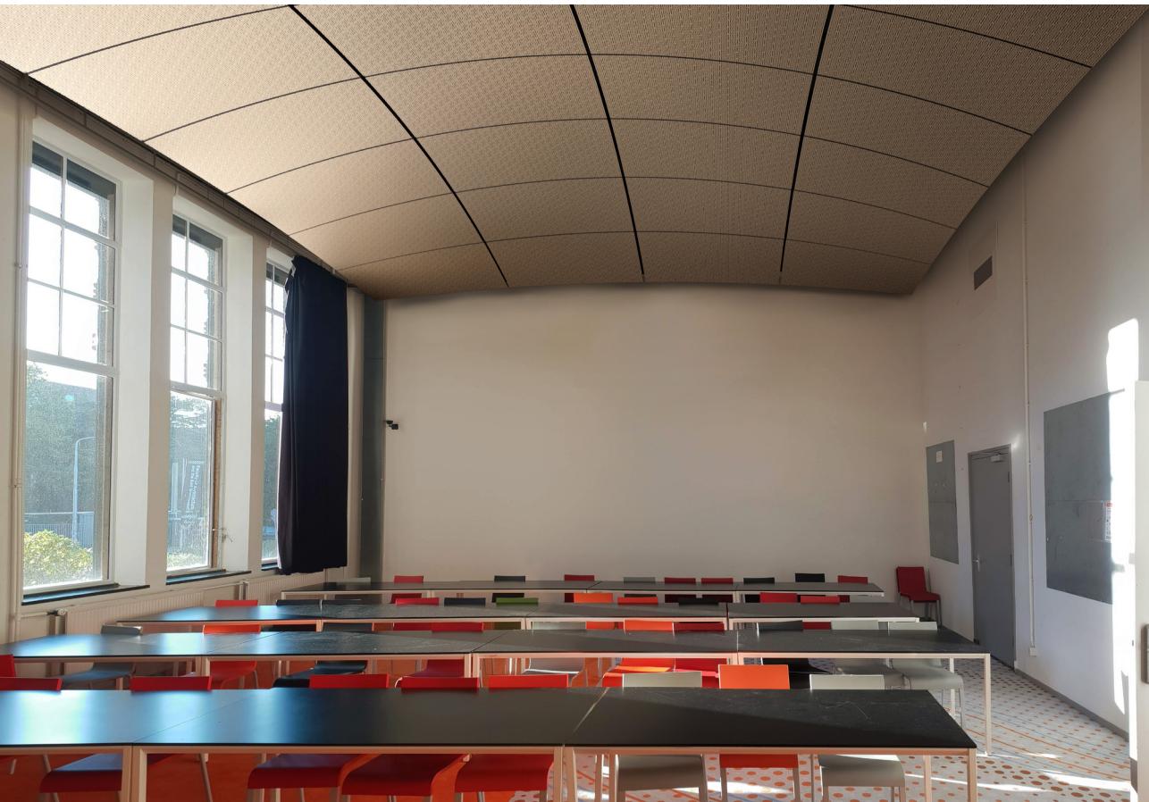
Figure 96. Acoustic panels applied in the lecture room, with a full parabolic surface.
