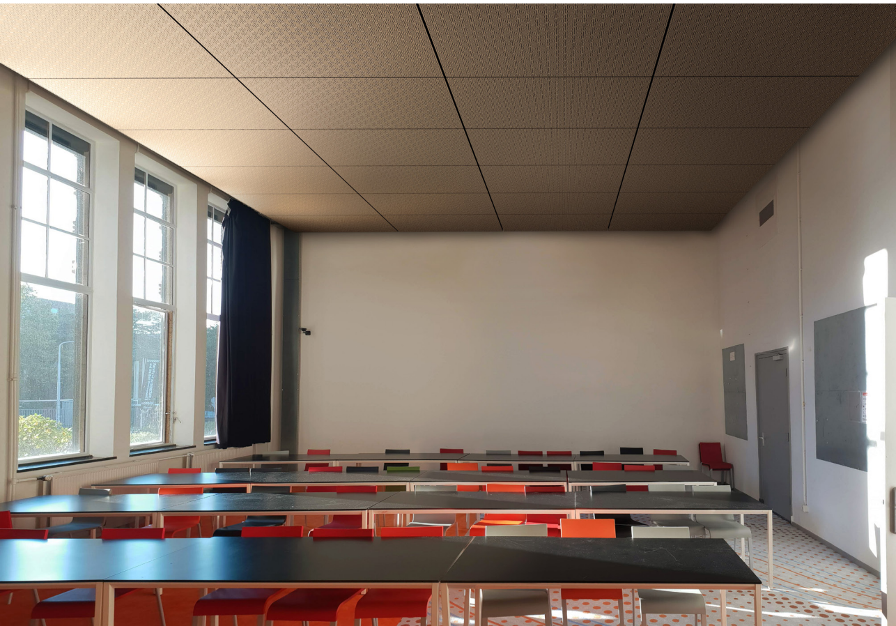
Figure 94. Acoustic panels applied in the lecture room, with a flat surface.
