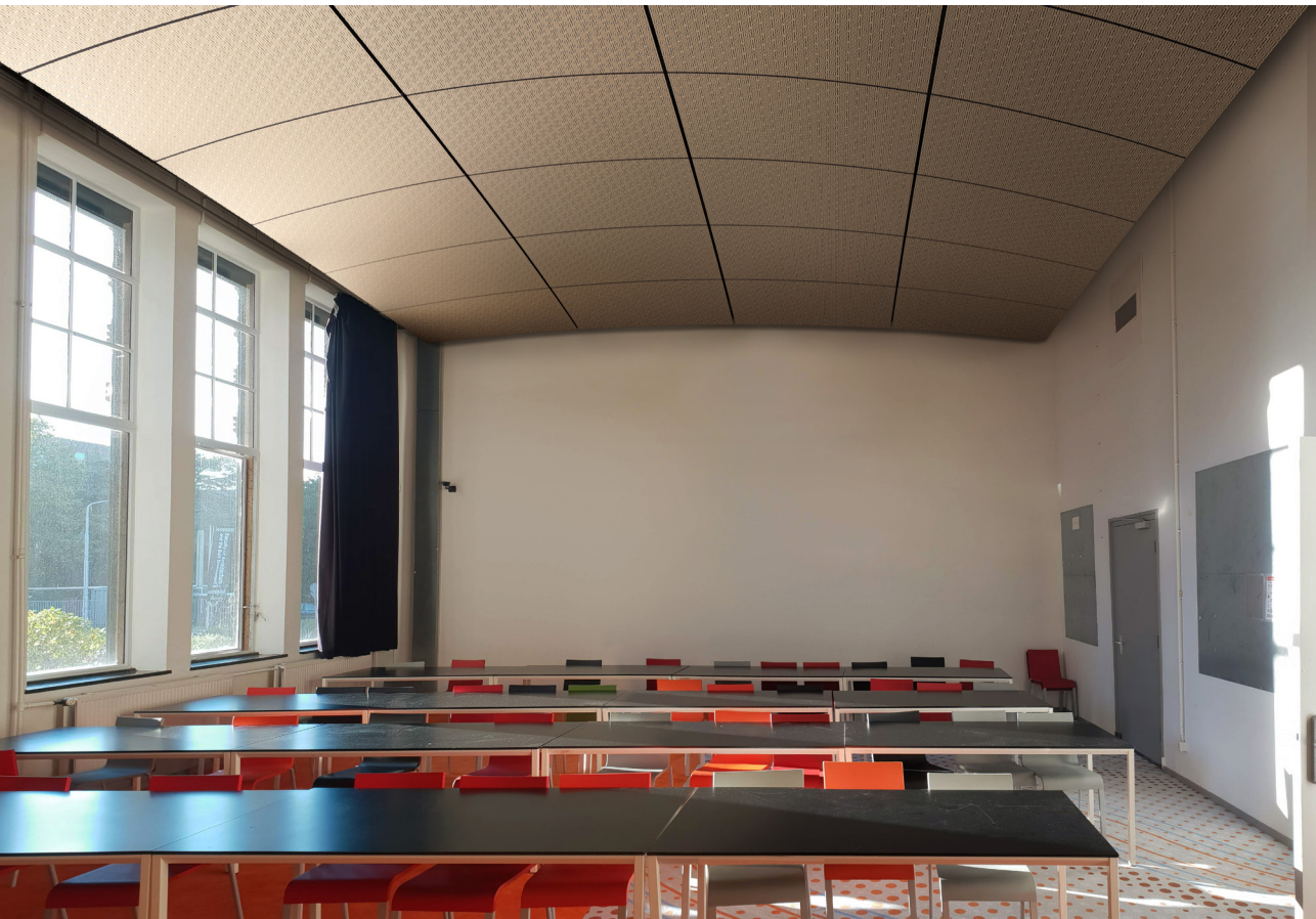
Figure 95. Acoustic panels applied in the lecture room, with a half parabolic surface.
