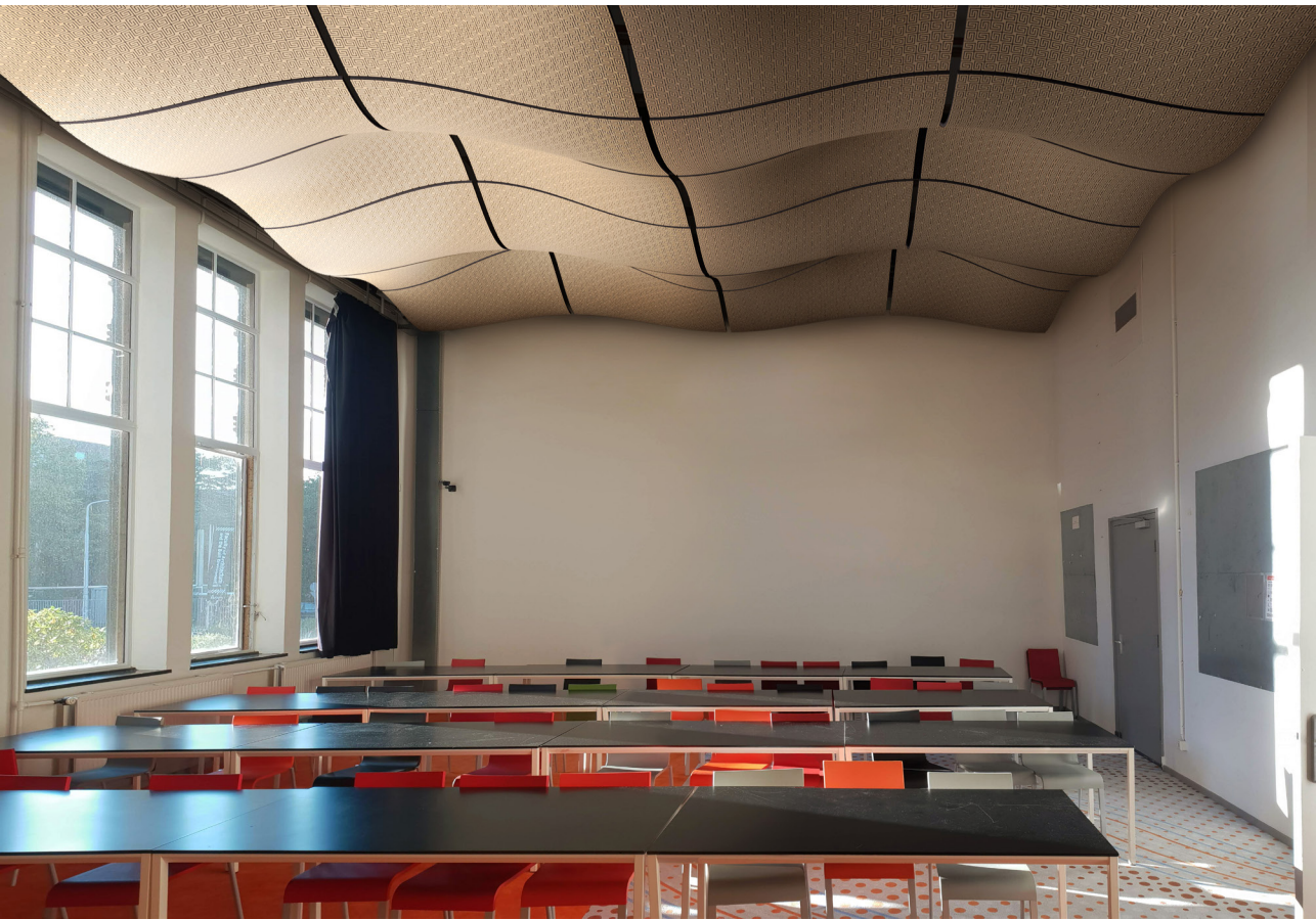
Figure 97. Acoustic panels applied in the lecture room, with a sinusoidal surface.
