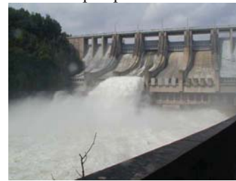
Fig. 9. Dams in the Cascade Barrier
