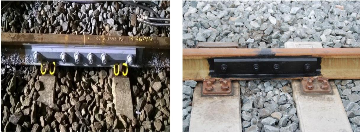
Figure 1.13: a) NRG-joint, b) ES joint
