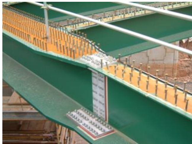
Figure 1.3 Headed stud connector on the left [7] Application of the headed stud on the right [9]
