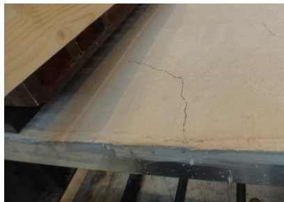
Figure H 14 Test Specimen 2, failure of the flange due to uneven loading due to imperfections top concrete layer.
