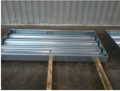
a) ComFlor75 sheets in place, including the joist shuttering.
