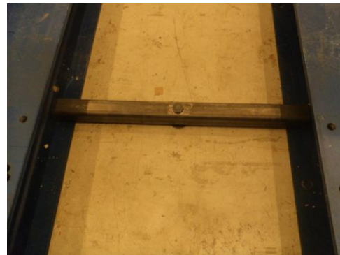
b) Anchorage of the two main beams to the 1200 mm thick concrete slab of the Stevin II laboratory.
