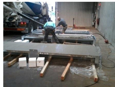
b) Flattening out of the top side after casting.
