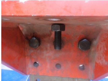
a) Nut below the support. To be twisted downwards.
