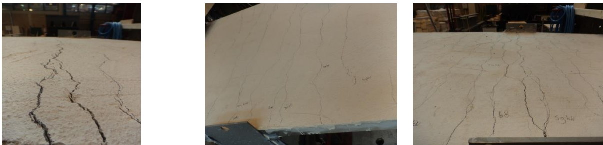
Figure H 17 Crack pattern of specimen 3, failure at the mid support, crack at 960mm from point of engagement.
