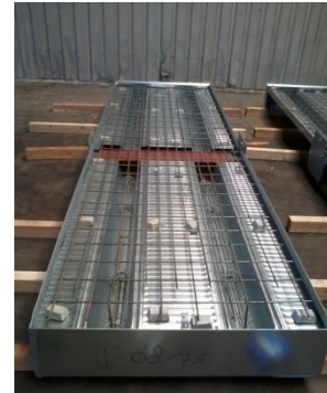
c) Reinforcement put in place in the ComFlor210 specimen.
