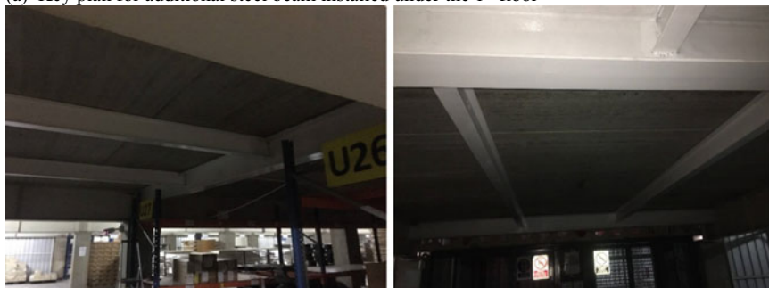
1st Floor after adding additional beams
