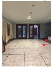
Travertine: travertine slabs as flooring in the vestibule, with red marble borders.
