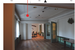
Plasterwork: plastered ceilings in dining rooms and hallways
