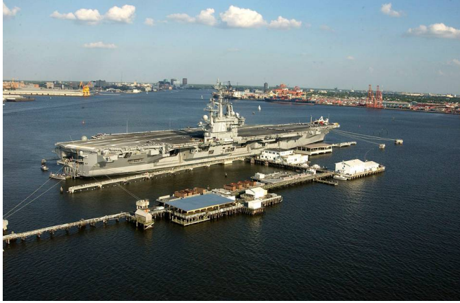
Figuur 1.4: The Lambert Point Deperming Facility located in the Elizabeth River just off Lambert's Point, Norfolk, Virginia, United States.
