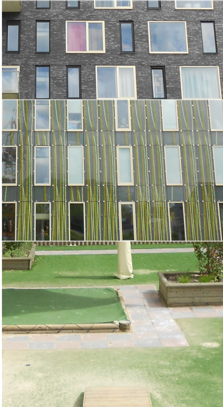
8 Django Building: Collective Space Facade & Paving Materials
