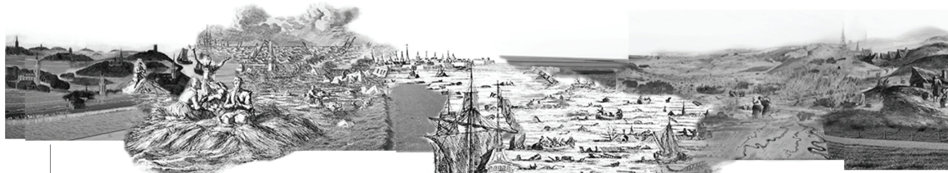
St. Elizabeth flooding 1421
