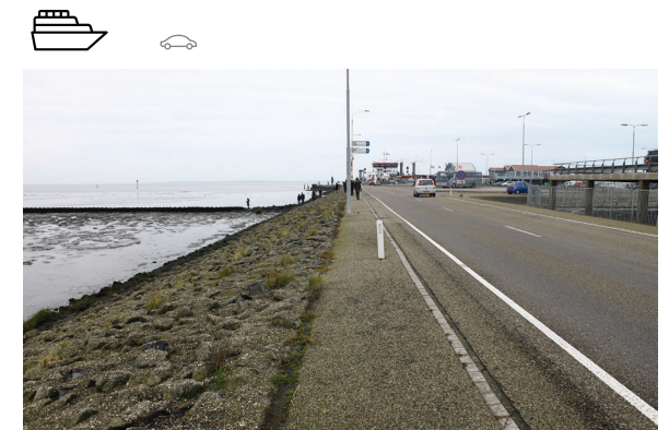
Pier, Holwerd (Own library)
