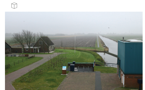
Pumping station, zwarte Haan (Own library)
