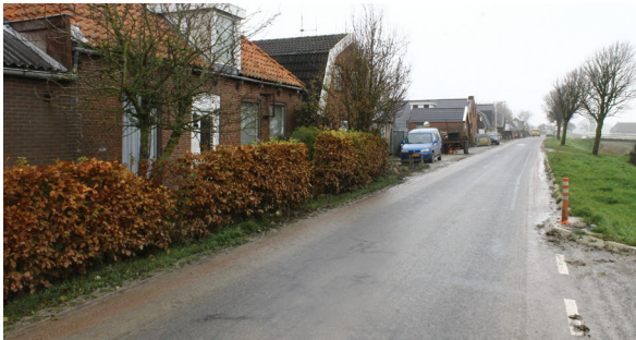
System of dikes, built area (Own library)
