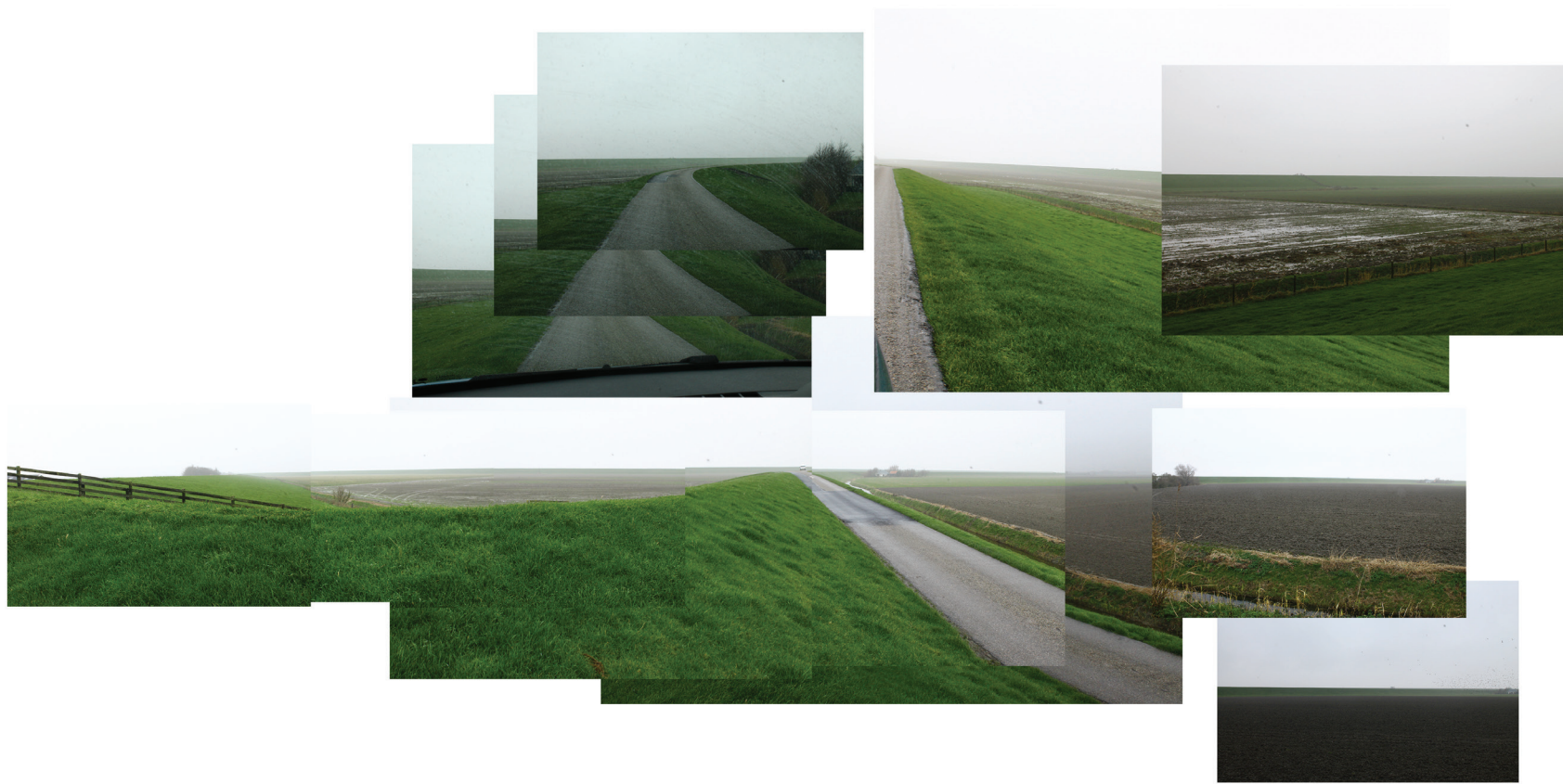
Materialization, use and experience 'being on' Omringdijk (Field trip, december 2017, Own library)
