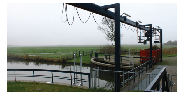
Viewing platform of pumping station landwards
