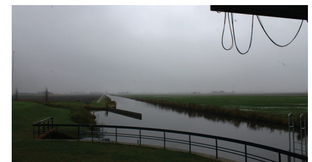
Straight inland ditch with small public path
