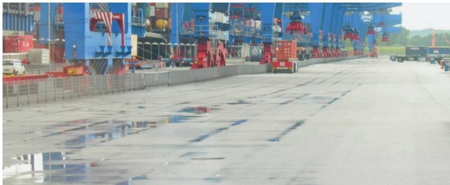
Figure 5.15 Ruts in pavement CTA terminal Hamburg
