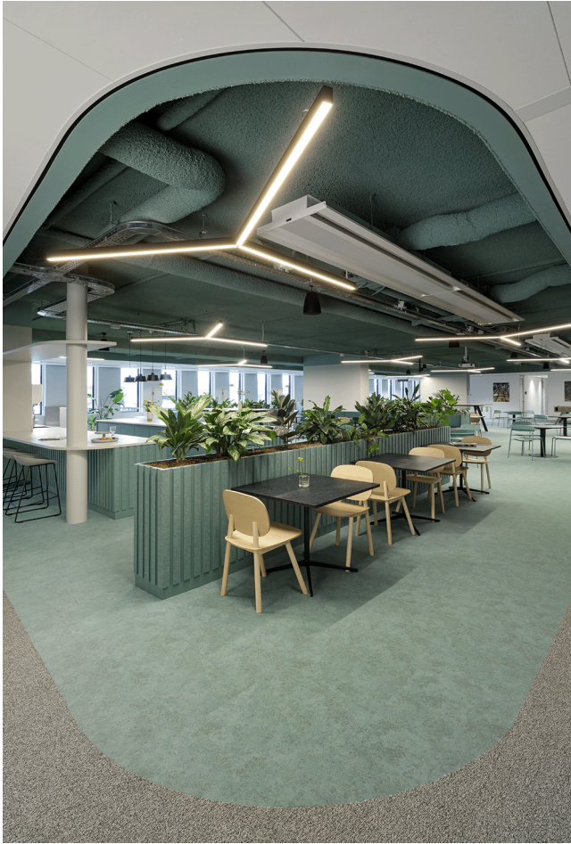
Figure 4.4.5. Acoustically sprayed ceiling (Colliers, 2024)
