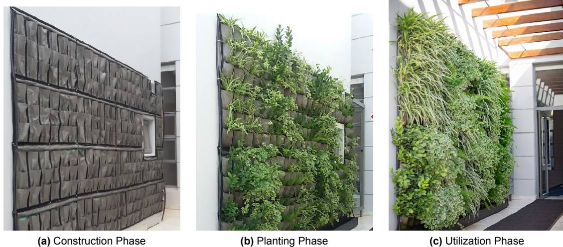
Figure 2.7: Pocket system (prod. Vertipockets ) by Living Green Walls in Cape Town, South Africa
