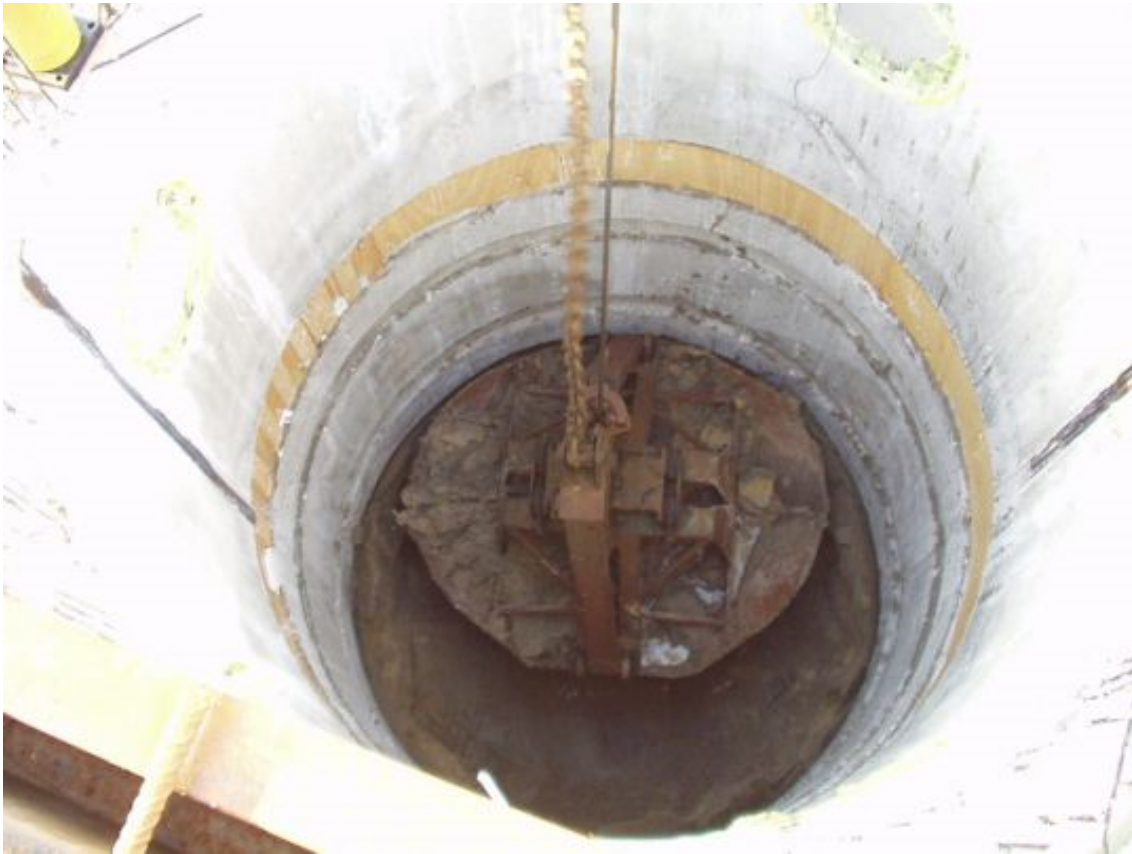
Figure D.1: Photo of the inside of an open caisson [VSE, 2014]
