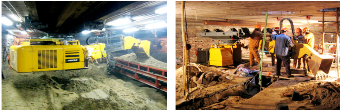
Figure 5.11: Automatic excavator inside the working chamber [Oraukia Tech, 2009]
