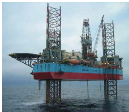
Figure 1.1: A jack-up rig showing its three enormous legs.
