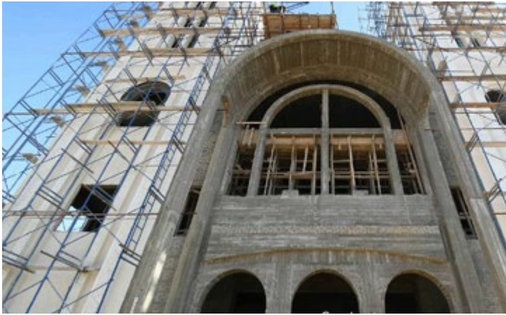
Figure 22: Construction photo of St. Mercurius church in New Cairo, showing the traditional structure. Retrieved from google maps
