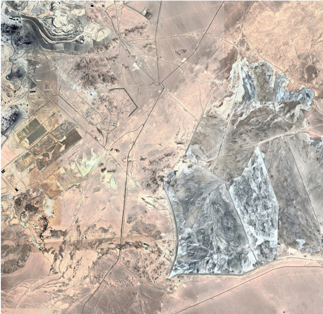
// 5 Satellite view on Chuquicamata Tailing Dam Tranque Talabre
