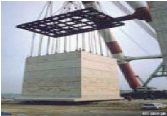
Figure 7.25 Handling of a caisson type quay wall in Japan
