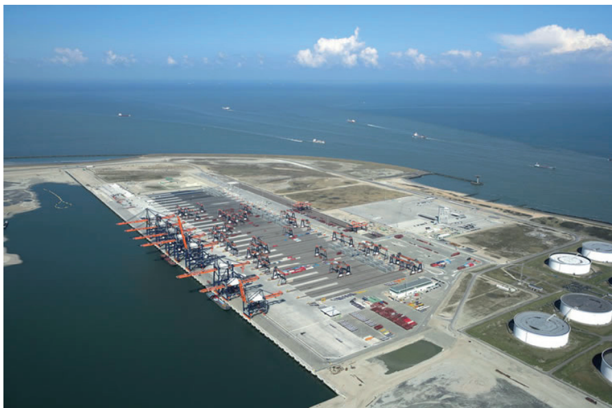
Figure 4.24: Maasvlakte 1, Rotterdam the construction of the Euromax terminal [HbR]
