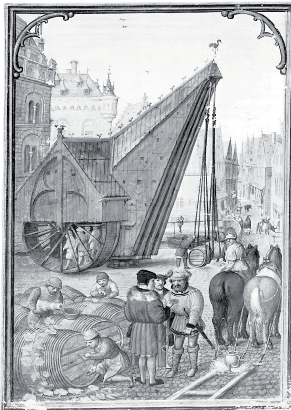
Figure 4.2: Treadmill in use in the port of Bruges [De Gijt et al 2003]
