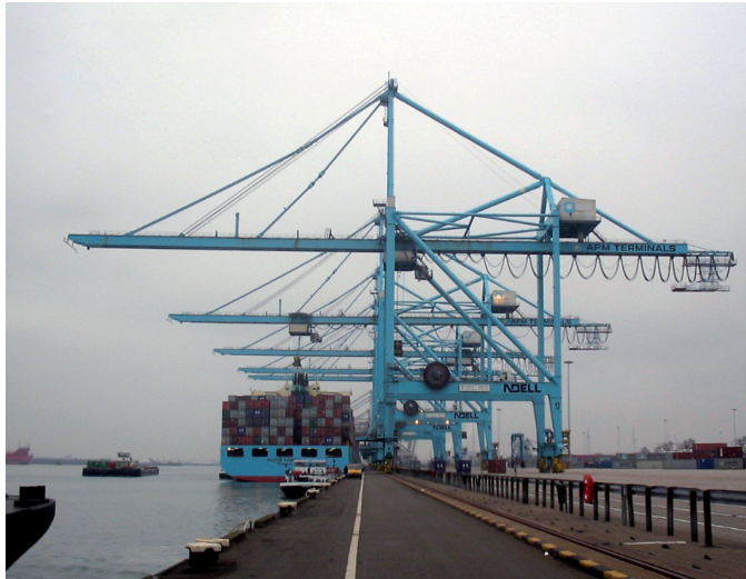
Figure 4.23: Container crane terminal Rotterdam [HbR]
