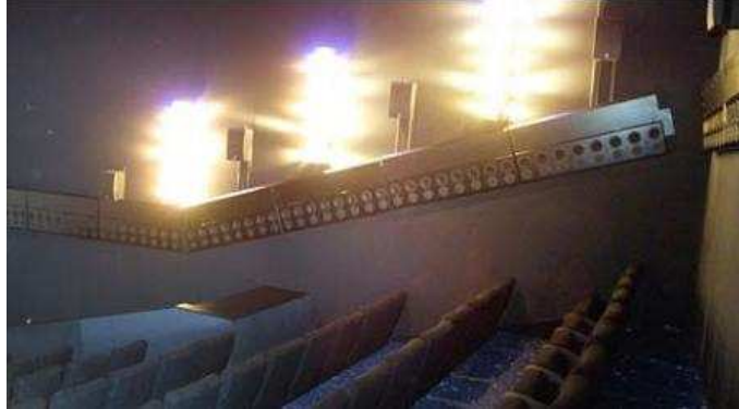
Figure 2.5: Cinema in Ilmenau, Germany that utilizes the WFS technique equipped with 192 loudspeakers.
