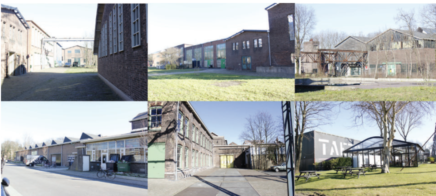
fig-4 : the first 5 images (anticlockwise) show the repetitive architecture, the last image on the bottom right shows a contrasting piece of architecture on the same site
