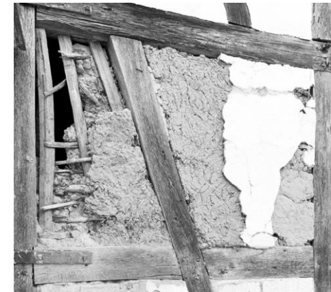
Traditional Clay-Timber Hybrid
