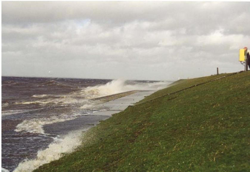
Cluster 1: *Rotterdamse Hoek* ('Rotterdam corner', named after the debris of the 1940 bombings of Rotterdam city, that were used for the construction of the dike between the towns of Urk and Lemmer)
