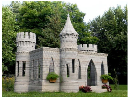
Fig. 2. 2: BigDelta project of a 3D printed castle [70]
