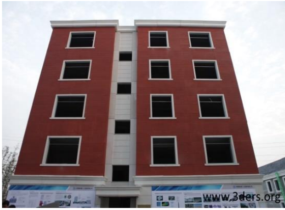
Fig. 2. 1: WinSun China build world's first tallest 3D printed apartment building [69]
