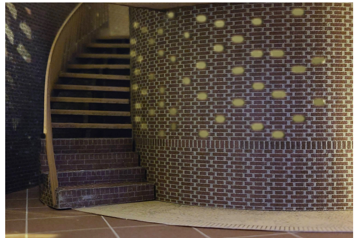
Brick expression: stairs up till 1 meter are brick and perforated wall connects interior
